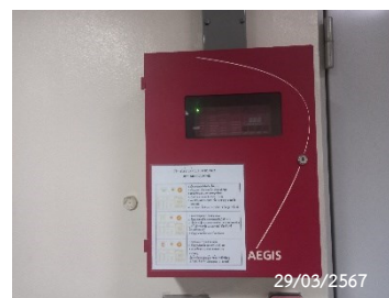
Fire Alarm Control Panel
